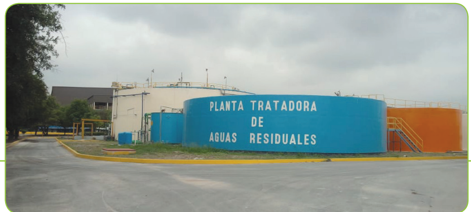
Our Escobedo, Mexico, assembly plant operates a zero-discharge wastewater treatment facility, pictured, which contributes to more efficient water use.
