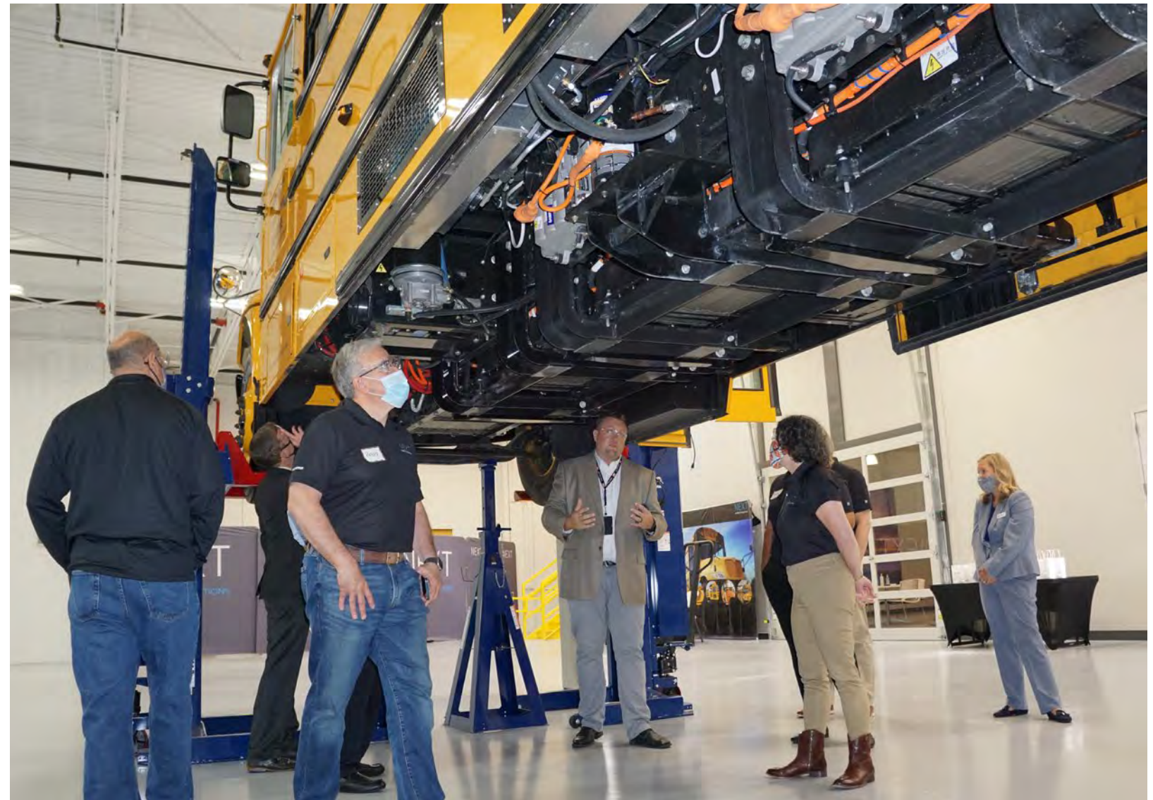
LEFT: INSTALLATION OF BATTERY PACKS AND ASSOCIATED COMPONENTS ON A CHASSIS OF AN ELECTRIC BUS AT TULSA, OKLAHOMA, BUS PLANT.
